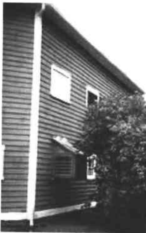
Installing a fan (successfully concealed here) for increased ventilation can be a successful low-tech substitute for air conditioning. Photo: Courtesy, Shelburne Village.
