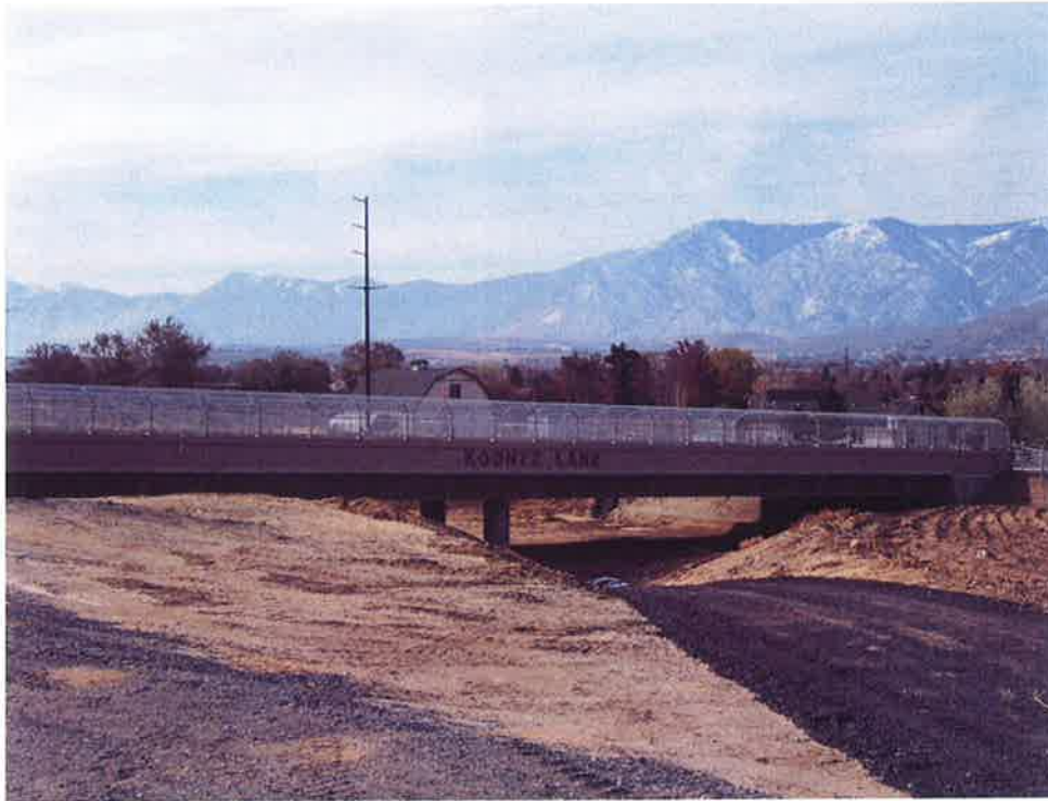
Koontz Lane Bridge
