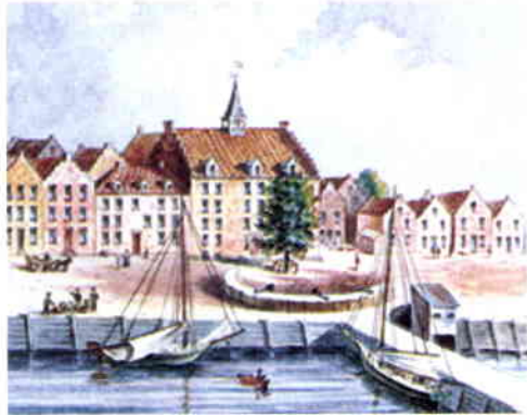
The tile roof on Stadt Huys (City Hall), New Amsterdam may have been imported, but by the time of its construction in 1641-42 tile was probably available from a tile yard up the Hudson in Rensselaerwyk. (Image courtesy of the Museum of the City of New York)
