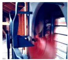
Installing ventilating fans can improve damp conditions or reduce cooling loads. Photo: NPS
