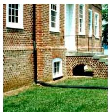
The owner used long black extender pipes to test a theory that it was faulty roof drainage causing the problem. Photo: NPS files.
