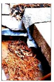
Debris will impede the normal flow of water from the roof's gutter and downspout system to the ground and result in moisture problems. Photo: NPS files.
