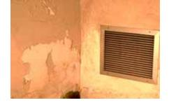
as a vapor, will seek to dissipate and equalize with adjacent spaces. Moisture can form on single-glazed windows in winter with exterior temperatures below 30°F and interior temperatures at 70°F with as little as 35% RH. Frequent condensation on interior window surfaces is an indication that moisture is migrating into exterior walls, which can cause long-term damage to historic
