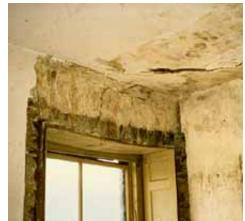
Damp interior plaster around windows generally indicates moisture has entered from the outside. Photo: NPS
