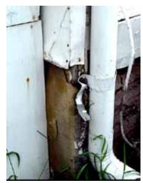
A clogged or broken downspout causes the water to pour directly into the ground. NPS files. Photo: NPS files
